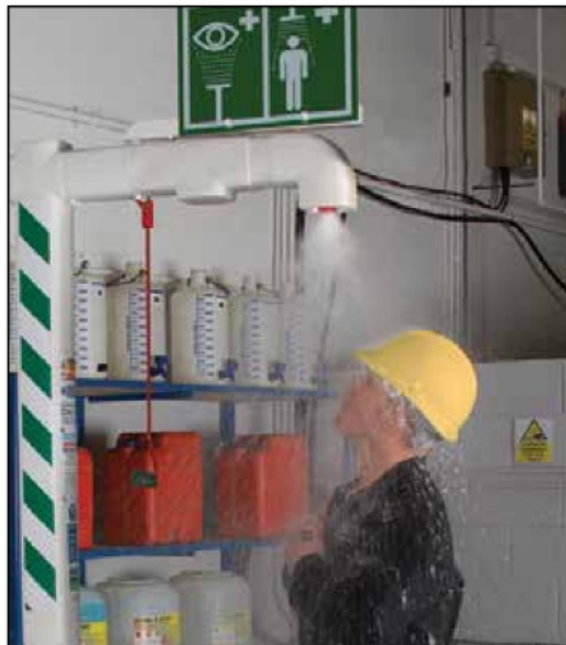
Heated and insulated for frost protection, use freeze protected showers in unheated indoor environments or outdoor cold climates.
