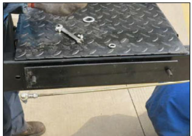
16. Route and mount the appropriate Cable(s) (Items # 94, 95, 96 & 97) to each Column Top Cap, while ensuring that the small, spring loaded Cable Pulley (Item # 41) is between the Cable and the Lock Ladder. This will allow the secondary slack cable lock to function properly. See Figure # 4 for Cable routing installation. **Note:** Make sure all Cables are properly routed around Cable Sheaves.
