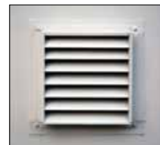
Vents with 3-hour fire damper
